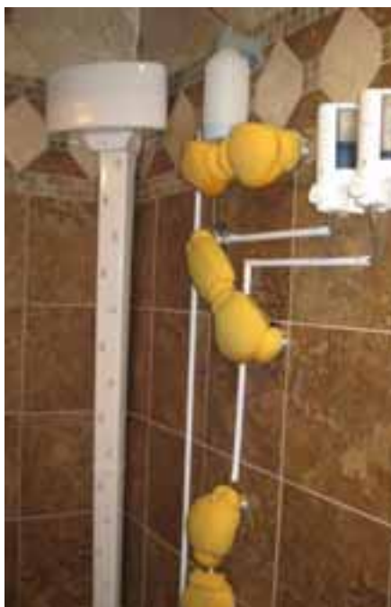
Shower modification with wall-mounted sponges for washing the body, soap dispensers controlled by a foot pedal, and a full-body dryer
